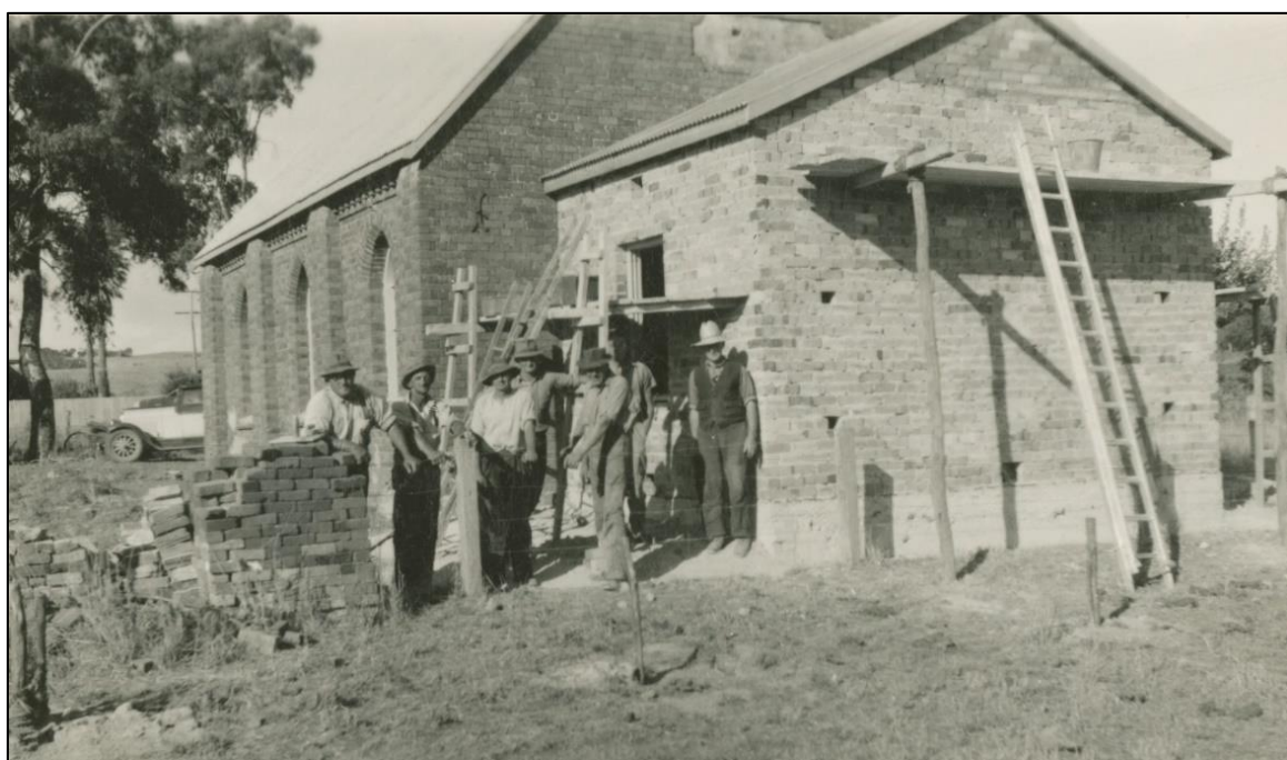
Original St Paul's Lutheran Church built 1858. Reclaimed and renovated to be used as a church hall in the 1950s. Builder Wilhelm Adolf Altmann on left , others to the right include: Ben Kramm, Eddie Rothe, and Edwin Braendler. Photo from the Lutheran Archives SA [P115 47 22910].
