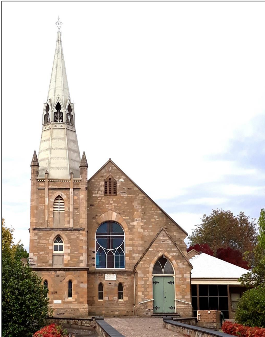
The current St Paul's Lutheran church in Hahndorf. Photo taken by the author in 2022.
